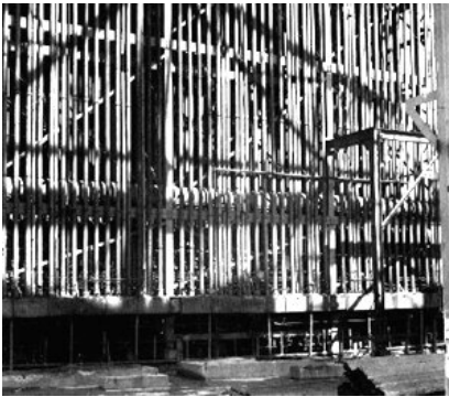
Liquid thermal diffusion uranium isotope separation columns, Philadelphia Navy Yard.
